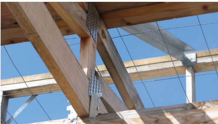
Photograph 12 – Parapet restrained back to roof with purpose designed metal angle
