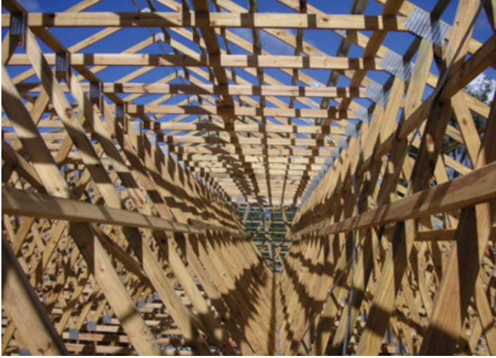
Photograph 8 – Web ties may be required for long webs. Check the specifications
