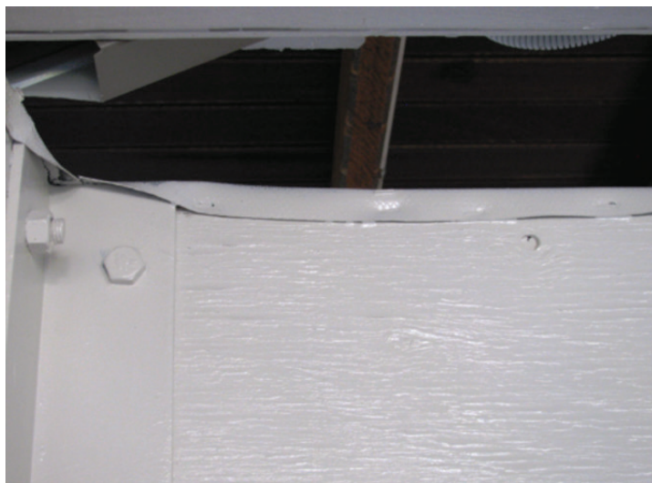
Photo 5: Flashing installed over H3 LVL beam under a deck.
