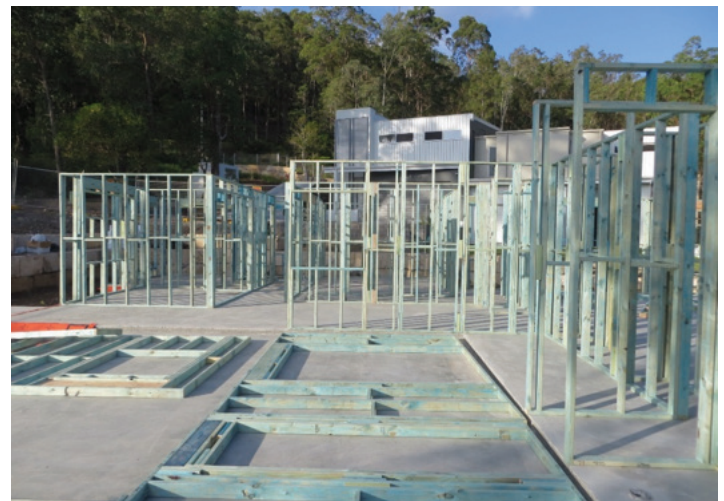
H2F termite treated structural softwood framing.
